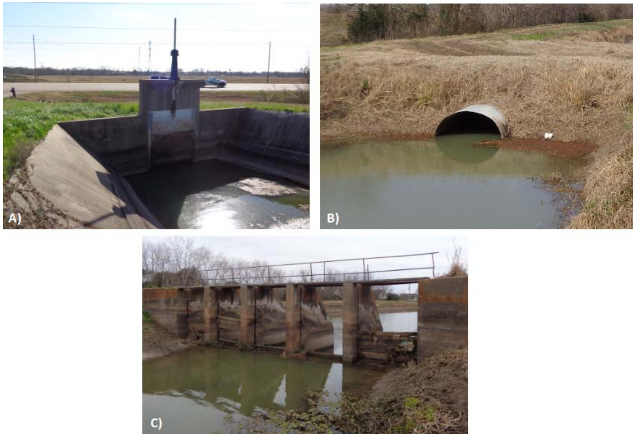
Figure 24 – Structures within the GCWA canal system – A) Gates, B) Culverts, and C) Check stations. Recording water levels at each structure would allow for the computation of flow past the structure as well as water stored in the canal section immediately upstream of the structure.
